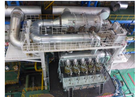
SCR-installation on WinGD field test vessel
