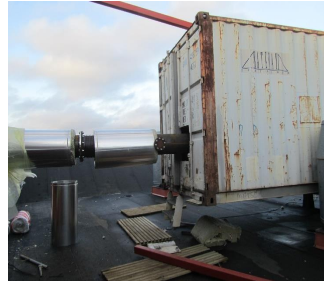
ESP + Cyclone container and inlet pipe during installation
