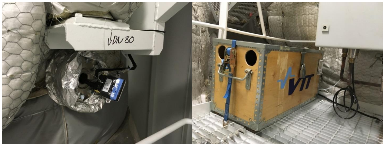
Figure 17. NH 3 sensor installation on ship trial 2. Sensor installed in the exhaust line on left hand side and accessory box for computer, power supply etc. on right hand side.
