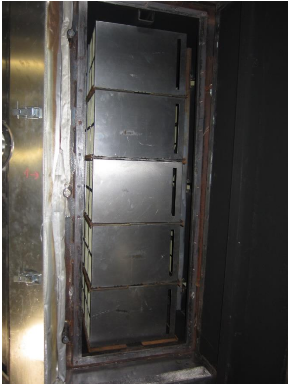
Figure 18 View inside the SC reactor showing the rectangular catalyst bricks
