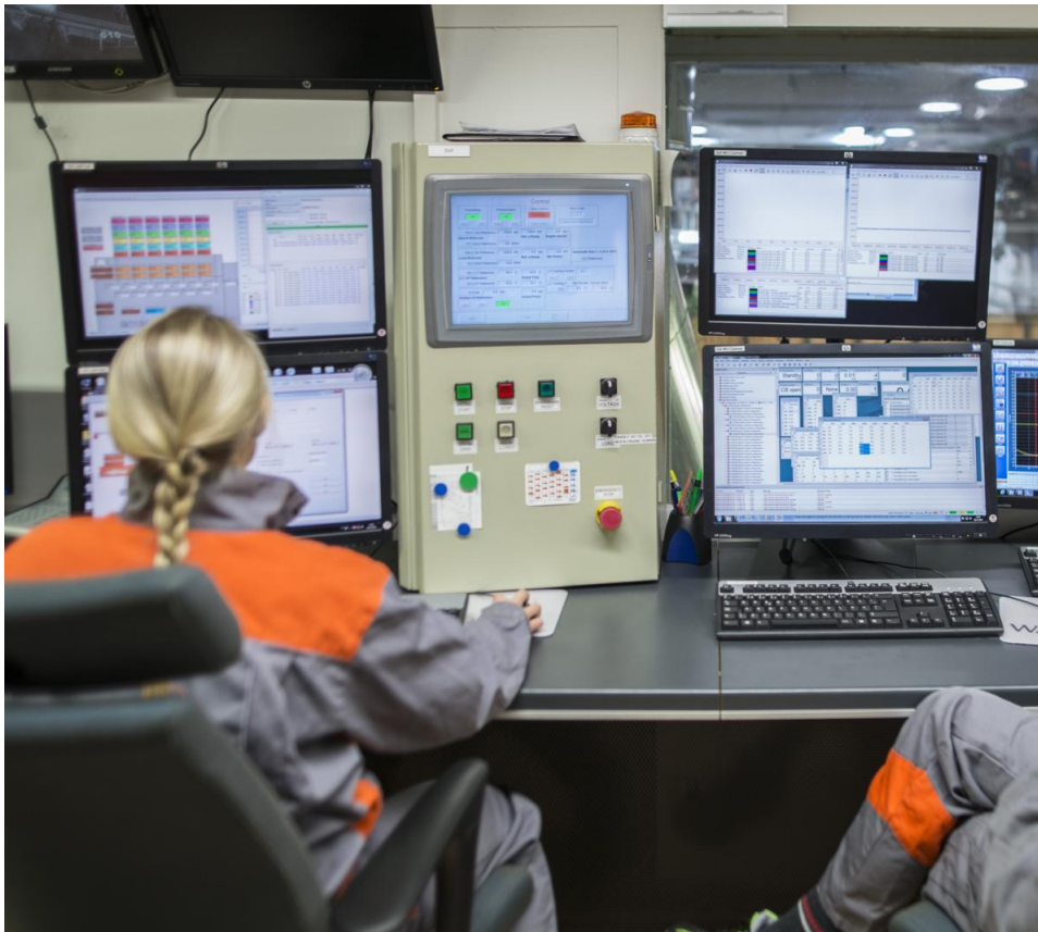
Figure 20: control room during testing
