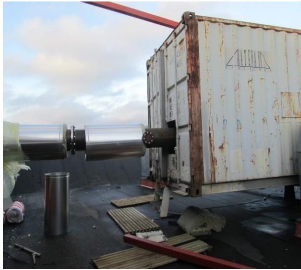
Figure 2: ESP + Cyclone container and inlet pipe during installation
