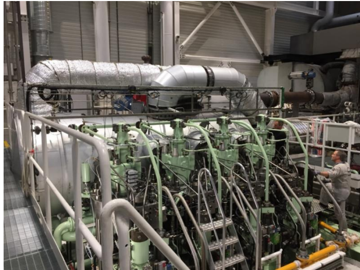
Figure 1 Integrated SCR receiver installed on a 4-cylinder 2-stroke R&D engine
