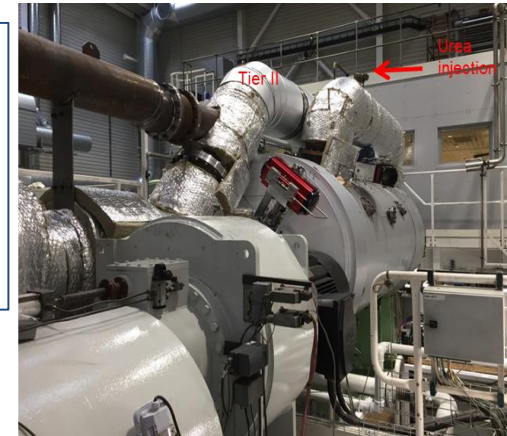
Engine Integrated SCR Installation on a 2 stroke 4 cylinder diesel engine.
