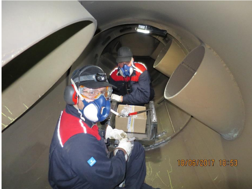
Installation of field test catalyst device in exhaust manifold
